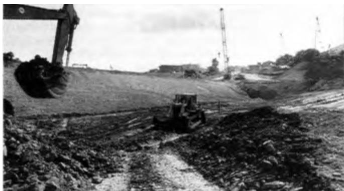
Linear cut-and-cover tunnel under construction at Holywell Coombe looking south-west.
