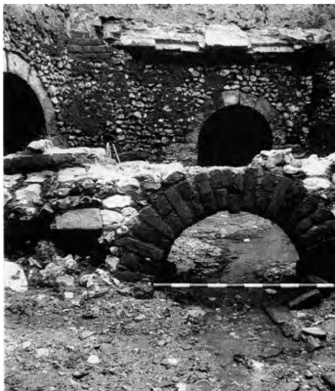
St Augustine's Conduit House; The summing foundation courses of the dividing wall with brick arch, tunnels in background. Looking north-east. Scale: 1m
